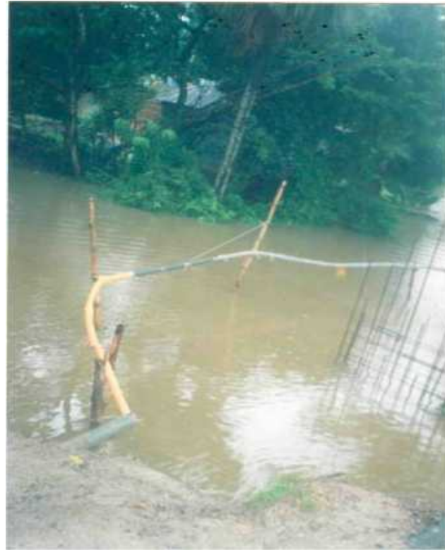
Flood damage to fiber optic link
