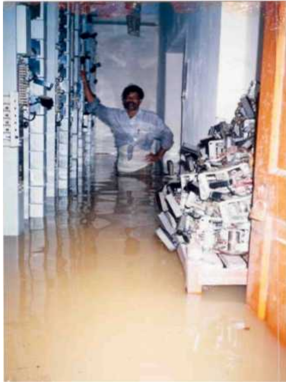
Flood damage to telephone exchange
